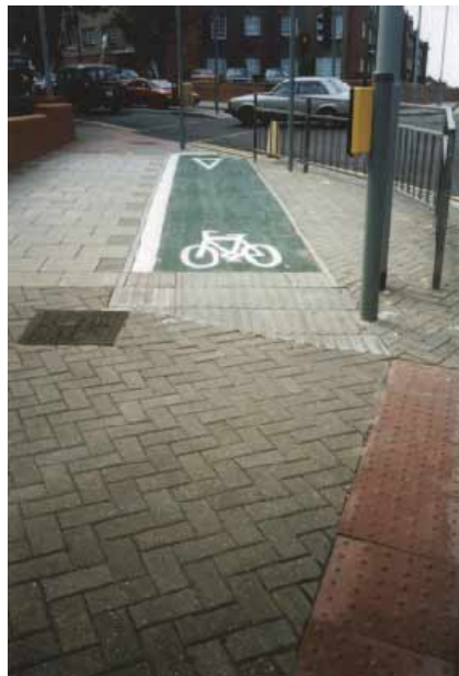
Above: Ribbed 'Tramline' tactile paving for cycle track - Sheepcote Road, Harrow
