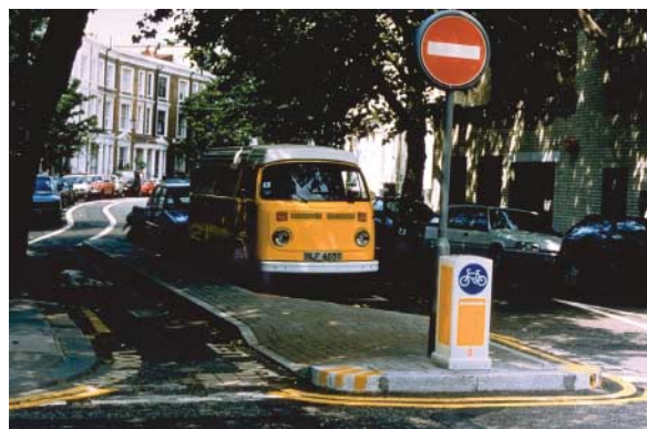
Below: Contra flow cycle lane outside parked vehicles - Kempford Gardens, Kensington
