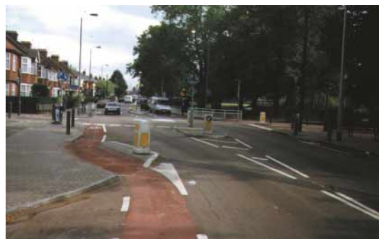
Above: Cycle bypass at entry to mini roundabout - Burntwood Lane Wandsworth
