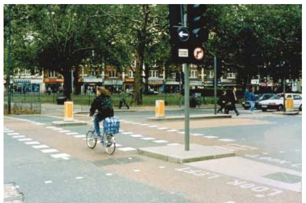
Above: Use of 'elephant feet' can help cyclists at complex junctions - Shepherds Bush
