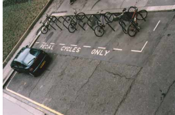
Above: Mastic Tarmac Surface - City of London
