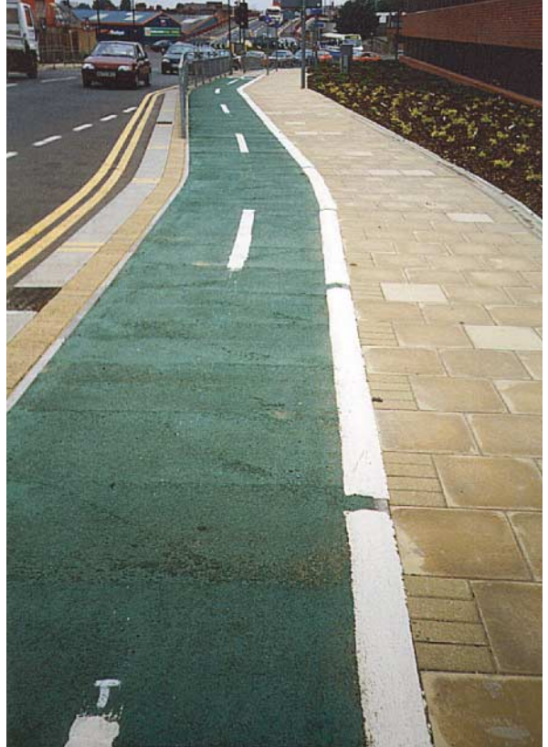
Above: White line segregation by means of revised line (1049.1) and with 500mm edge strip adjacent to carriageway - Wealdstone Harrow
