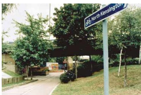
Above: Bridge over cycle path - North Kensington
