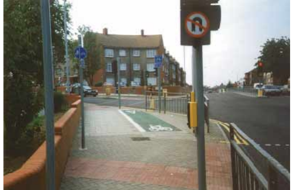
Above: Tactile paving should be simple and logical - Sheepcote Road, Harrow
