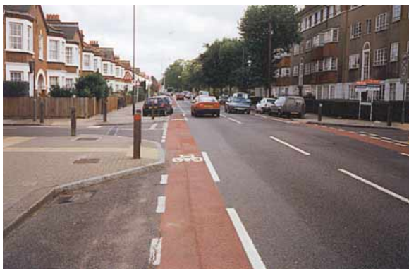
Above: Kerb build out at junctions, with ACL - Burntwood Lane, Wandsworth
