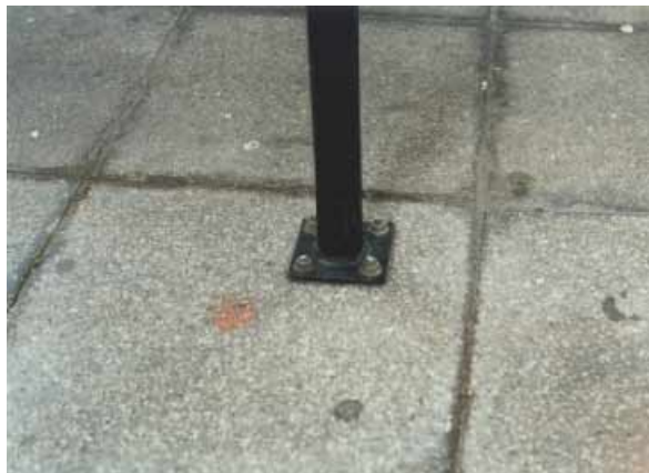
Above: Sheffield stand bolted down
