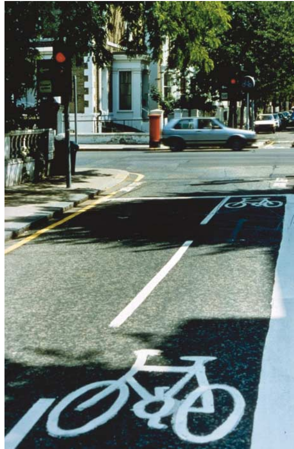
Above: Offside cycle approach to cycle gap in no-entry road - Lower Addison Road, Kensington
