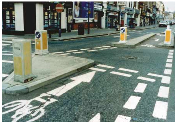
Above: Unsignalled cycle crossing – King Street, Hammersmith
