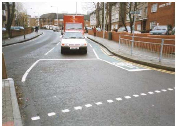
Above: Advanced Stop Line where cyclists do not need to turn right - Gayton Road, Harrow
