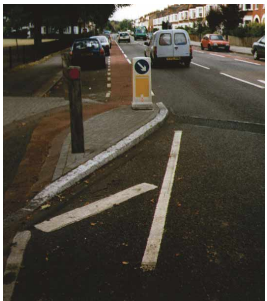
Above: Cycle bypass at throttle leading onto ACL - Burntwood Lane, Wandsworth
