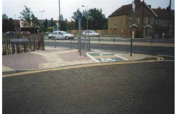
Above: Buff coloured blister with contrasting surrounding surface - George Gange Way, Harrow
