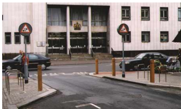
Above: Stainless Steel Stands on Build-Outs - Wandsworth
