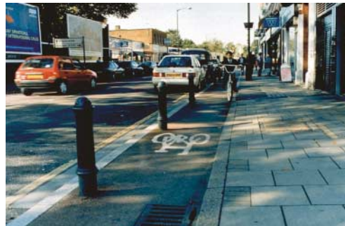
Above: Half kerb between footway and cycle track (contra-flow cycle movement) - Kingston
