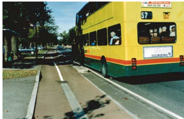
Bus stop boarding island
