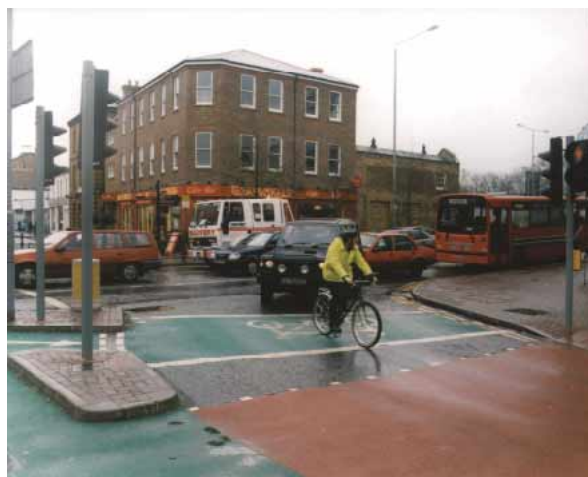
Above: Advance stop line with side entry - Eden Street, Kingston
