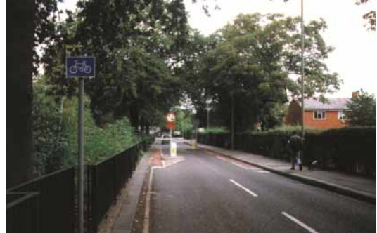
Above: Chicane with cycle bypass at throttle leading onto ACL - Aboyne Road, Wandsworth
