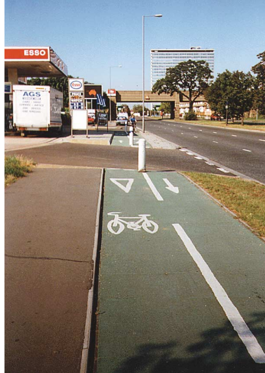
Above: segregation by level - Tolworth, Kingston
