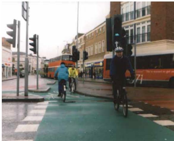
Above: Parallel crossing leading to junction island - Eden Street, Kingston
