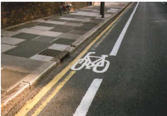
Above: Side entry gullies
