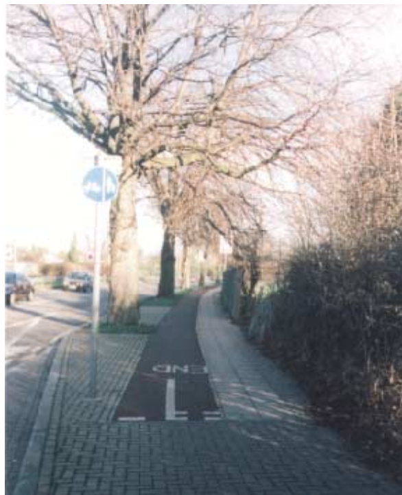
Above: Surface treatment and texture changes - Gt. Cambridge Road, Enfield
