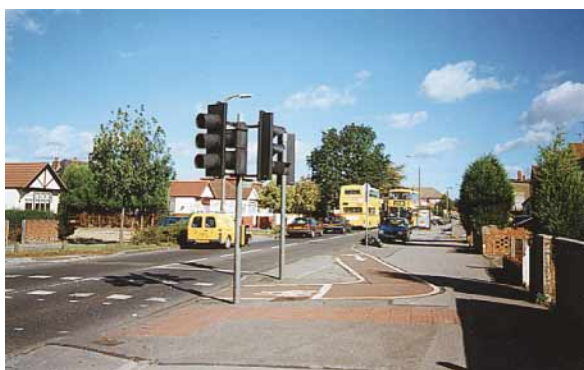
Above: Jug handle at Toucan to provide a right turn - Southend Road, Havering
