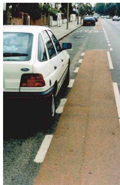
Above: Advisory cycle lane discontinued at bus stop
