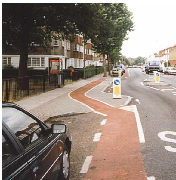
Above: Entry slip preceded by cycle lane to by-pass chicane - Earlsfield, Wandsworth
