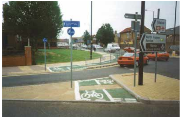
Above: Ribbed tramline tactile set back from kerbline - George Gange Way, Harrow
