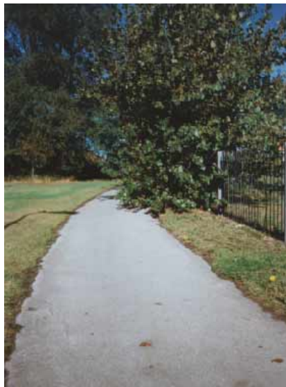
Above: Poor lighting and obstruction.
